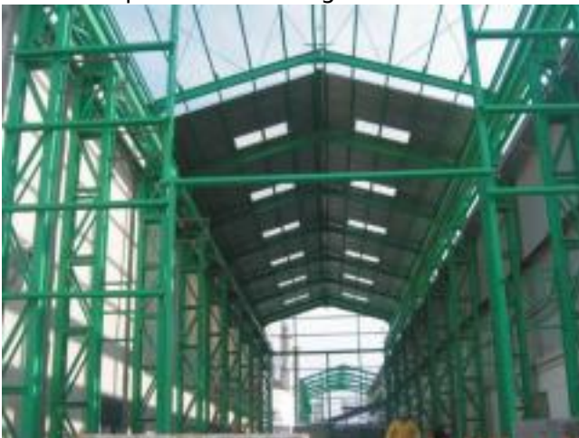
Erection of peb and sheeting works
