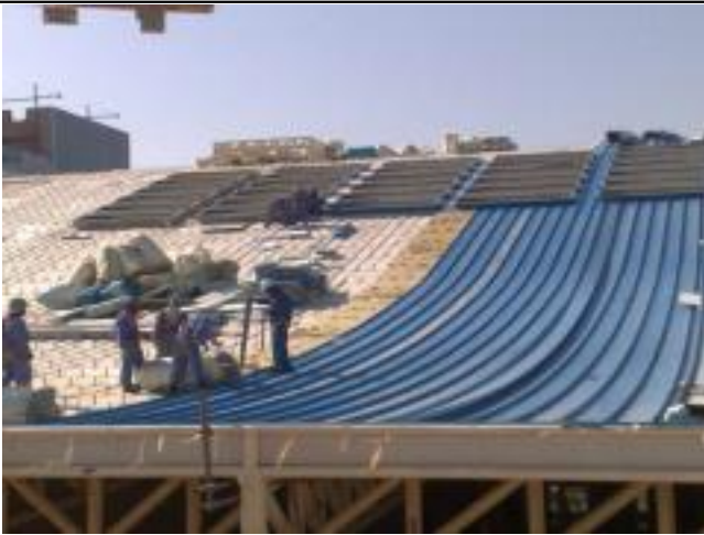
Cladding Roof
