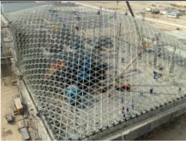
Space Frame Erection-Swege Treatment Plant Mesaieed
