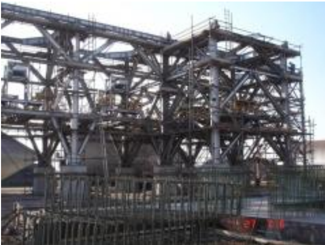
Pre-Fab & Erect Communication Towers
